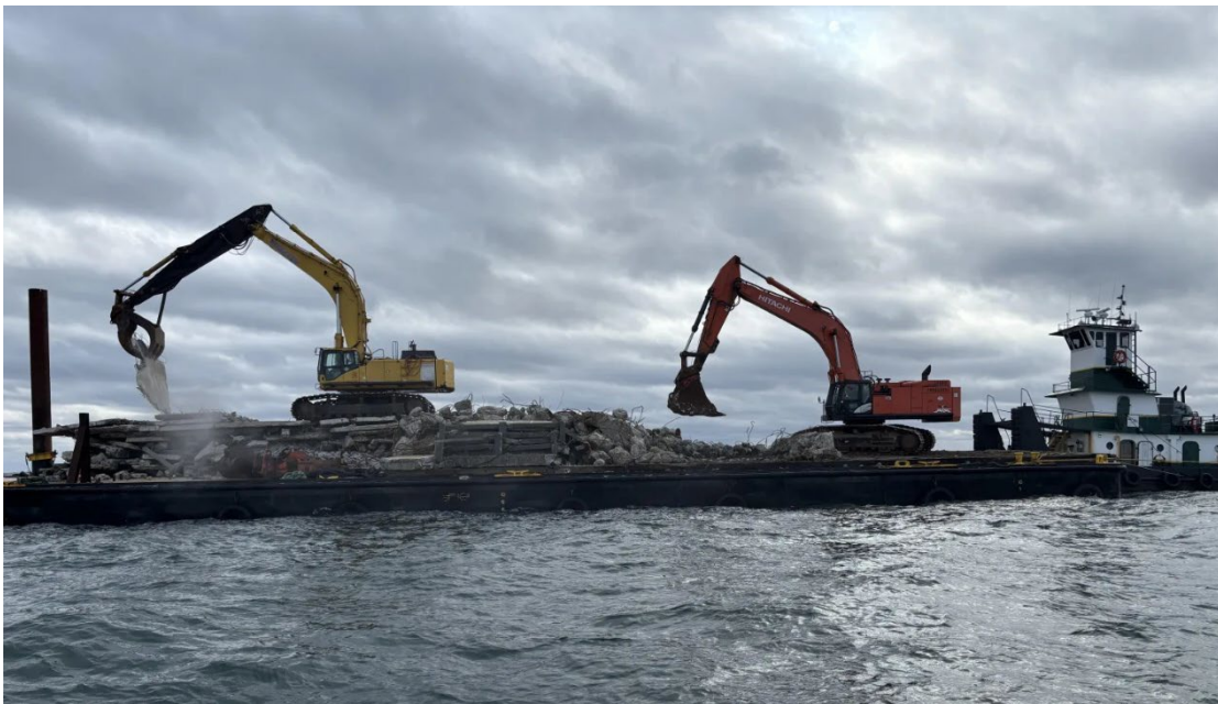
The tugboat and barge outfitted with cranes used to transport the material out the Shrewsbury River and deploy it on the Sandy Hook Reef. (Photo courtesy of Chuck Casagrande)
