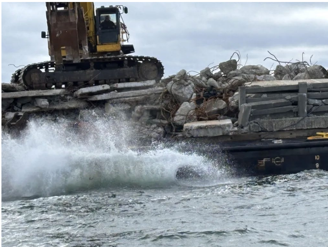
Water splashes as a big chunk of concrete is dropped onto the Garden State Reef.
